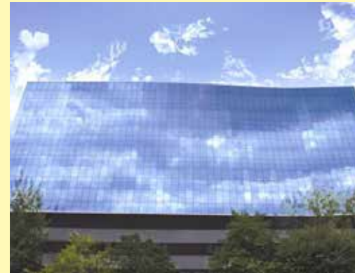
GODREJ ETERNIA SHIVAJI NAGAR, PUNE
